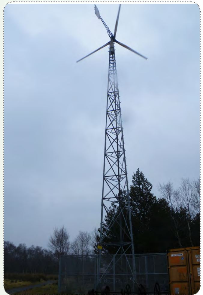
Wind turbine and secured area around it.
